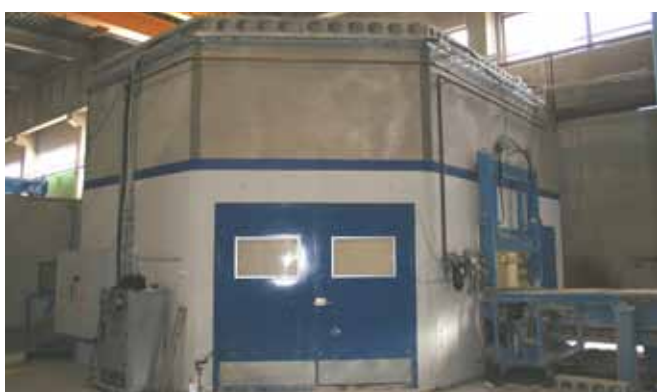
CutMaster sawing bunker.
